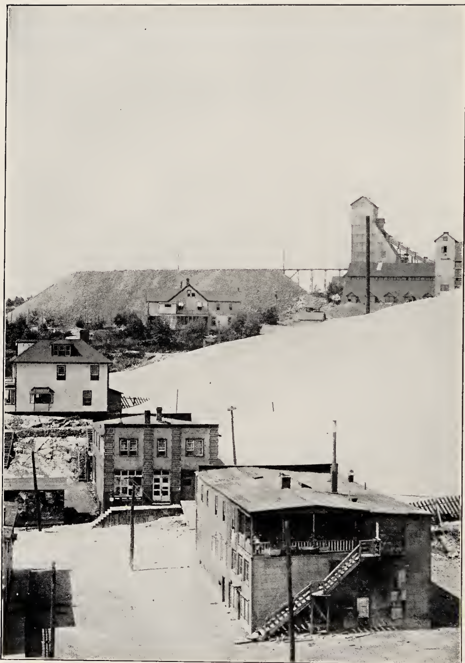
Since their discovery in 1903, the Cobalt mines have yielded silver bullion worth more than $200,000,000. These huge piles of tailings were formerly thrown away as waste. They are now being worked over again at a profit.
